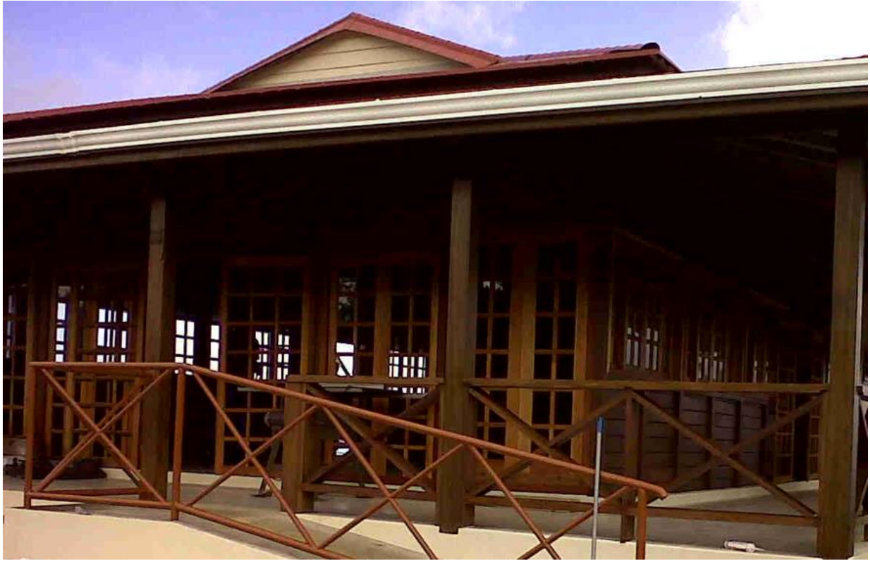
Varnish finish to be achieved at Bloody Bay Rest Stop – see item 3.2
